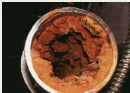
Localized Corrosion - A good example showing particulate deposits settling along the inside of the pipe, which will produce deep deposit pitting.
