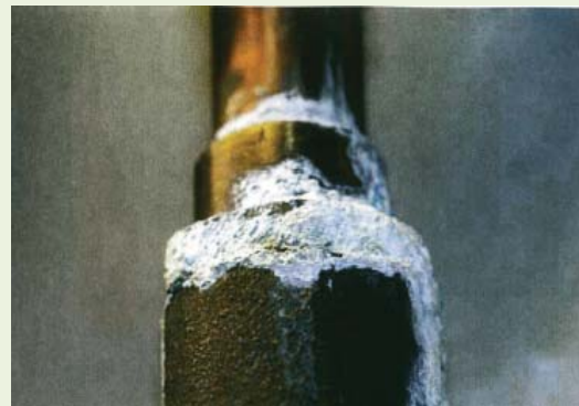
Galvanic Corrosion - An extremely common problem. A combination of water penetration and galvanic activity causing pipe deterioration.
